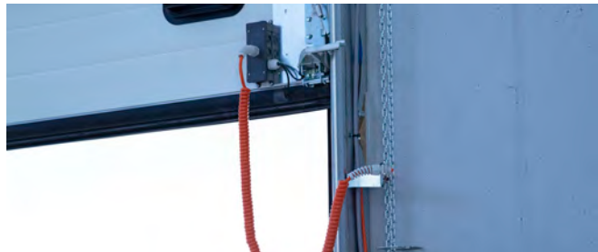
Cable break and spring break safety device
