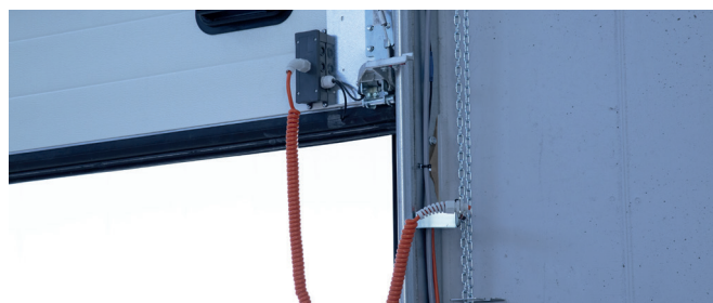
Cable break and spring break safety device
