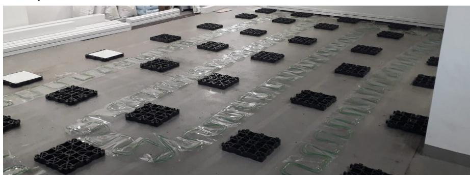
A heating mat controlled by thermostat from the electric panel can be installed between the rows of plates. This ensures a constant temperature below the floor panels to prevent dew point from being reached.
