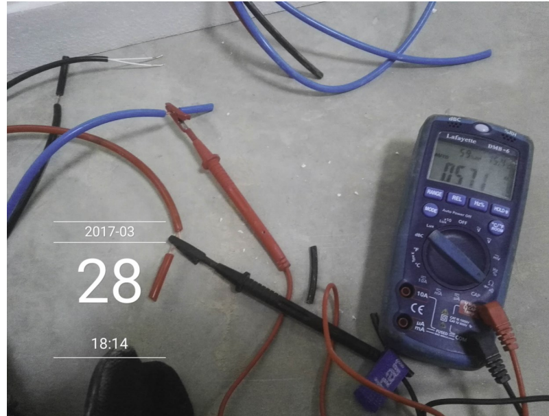
Reserve heating (blue-red cables)
